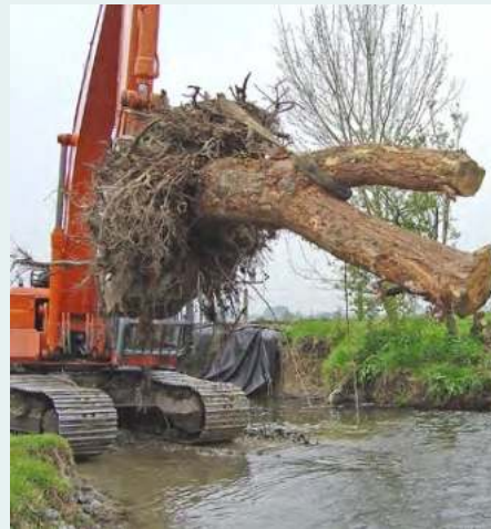
2. Moving root into position
