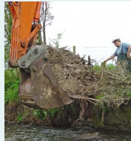
3. Installing Root Wad
