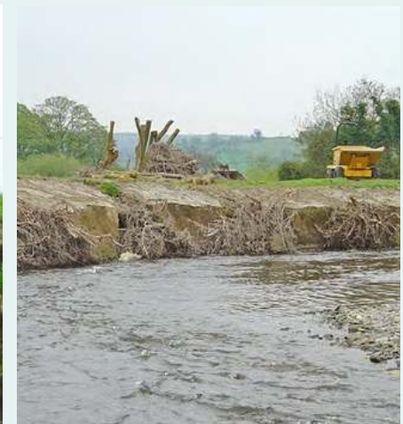
4. Right after installation
